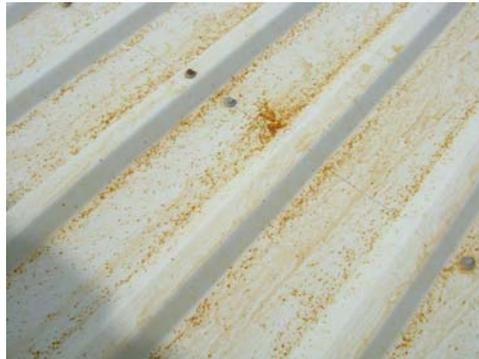
*Fig.1 Rusted speckles from metal filings that were sprayed across the sheet by cutting with an angle grinder*
