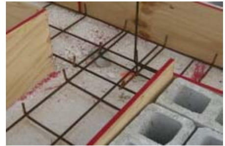
Typical Spaced at 12" Centres
